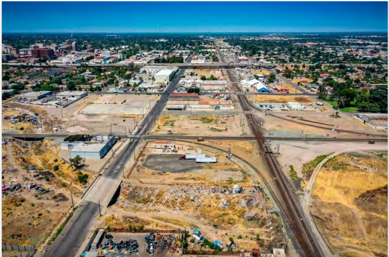
Two major rail lines cross at the Stockton Diamond, the most congested rail junction in California. A planned overpass and related upgrades got part of their funding in September 2020. SAN JOAQUIN REGIONAL RAIL COMMISSION
